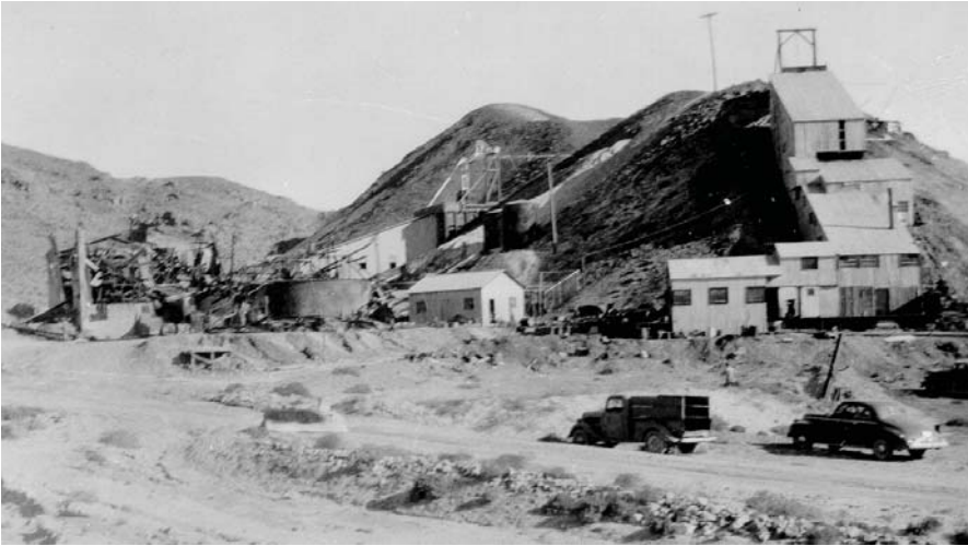
“The Black Mammoth Mill burned down in 1940 leaving only the E.L. Cord Mill operating in the district until World War II shut down the gold mines.” The remains of the Black Mammoth Mill in 1941. (Photograph courtesy of Gerry Cooper.)
